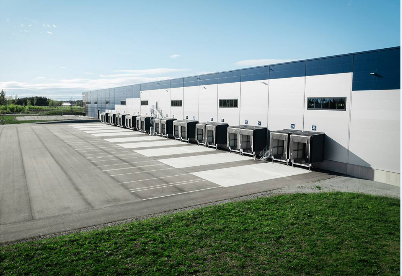
Loading Docks: External view of the docking facilities.
