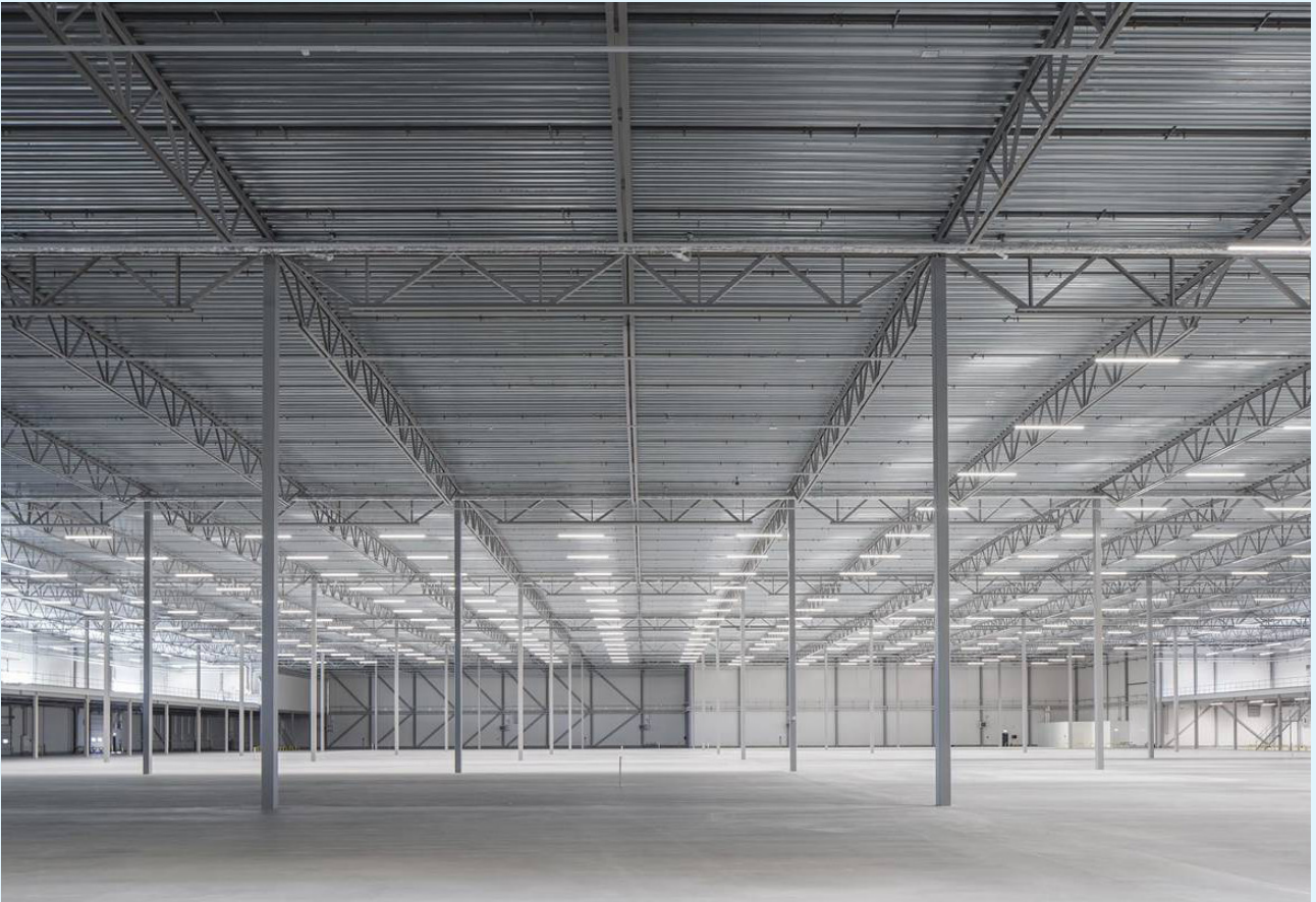
Interior: Warehouse space with 12-meter clear height.
