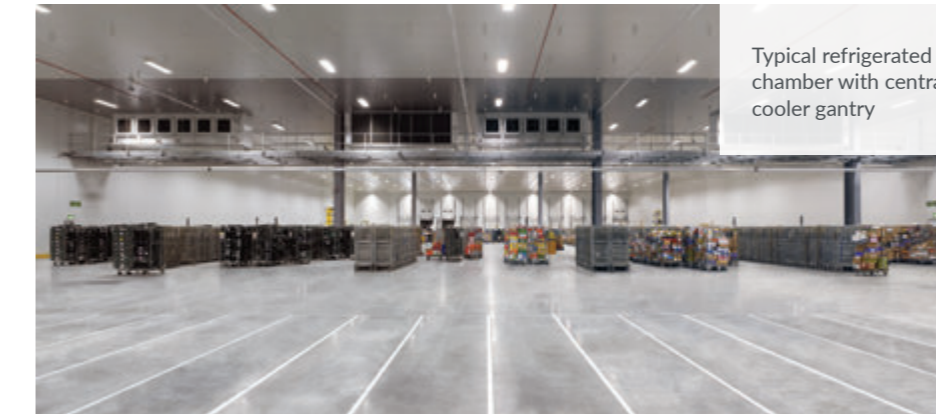
Typical roof void showing sprinklers and insulation panel suspension system
