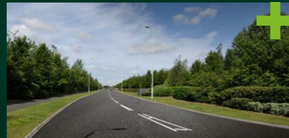
Maintained private roads
