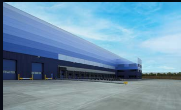
50m yard depth and suitable for 44 tonne HGV traffic, ensuring quality and durability.
