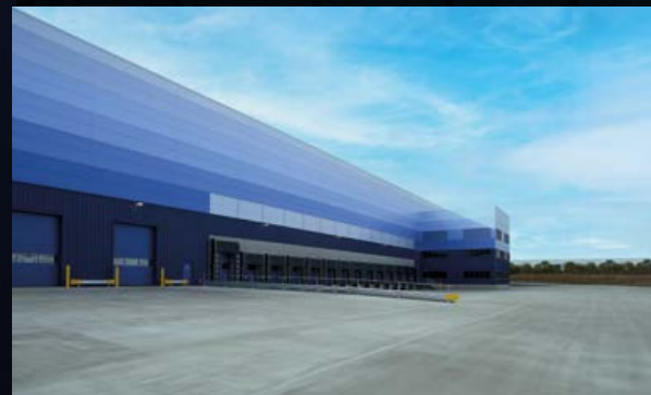
50m yard depth and suitable for 44 tonne HGV traffic, ensuring quality and durability.
