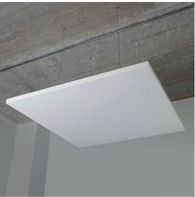
C1 - Exposed ceiling arrangement with exposed services and hanging lights. Ceiling areas to be formed with Ecophon Solo Rectangle Acoustic Ceiling Baffles 2400x1200, 2400x600, 1800x1200 or 1800/2400x100 (Special cut)
